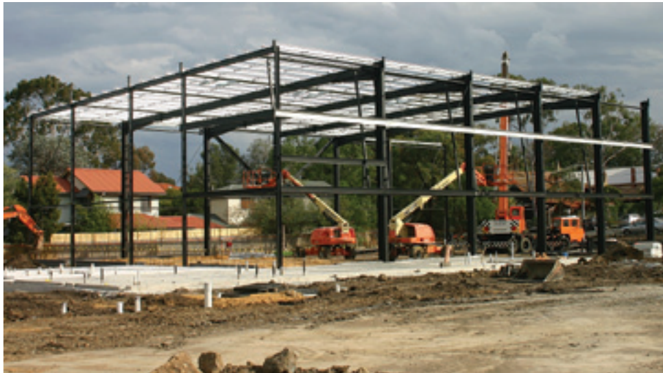
The Multi-Purpose building under construction
